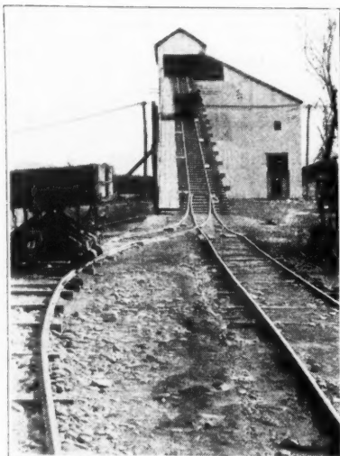
The Trestle and Track to The Preliminary Crushing Plant
